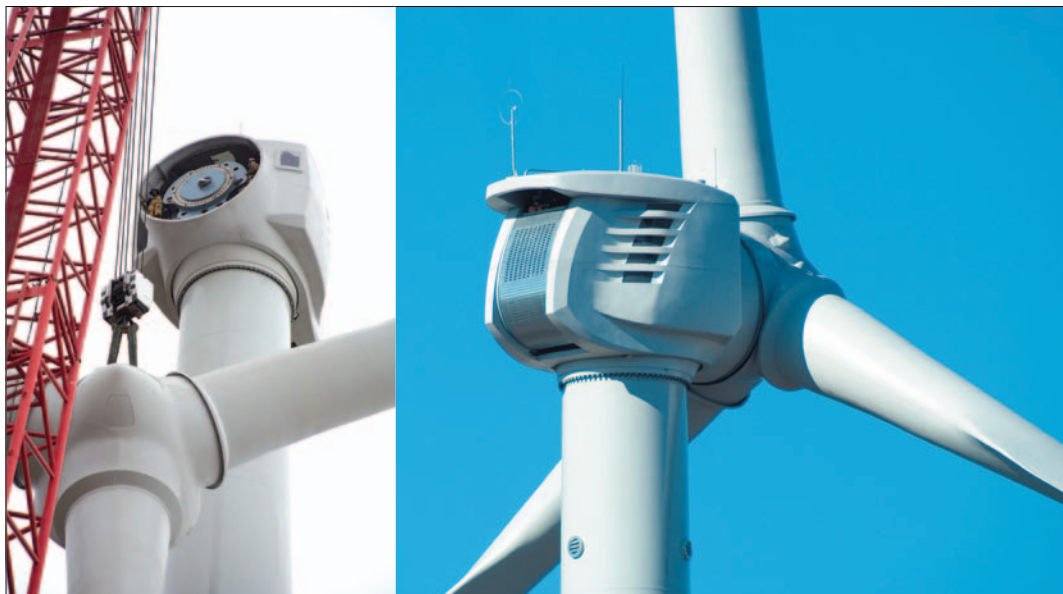
Behemoths like this Clipper Windpower 100MW Endeavor (left) turbine installation in Iowa and the 2.5MW Liberty—the largest in the U.S.—require like-sized components, particularly gearboxes, rotors and bearings. Photos courtesy Clipper Windpower.
