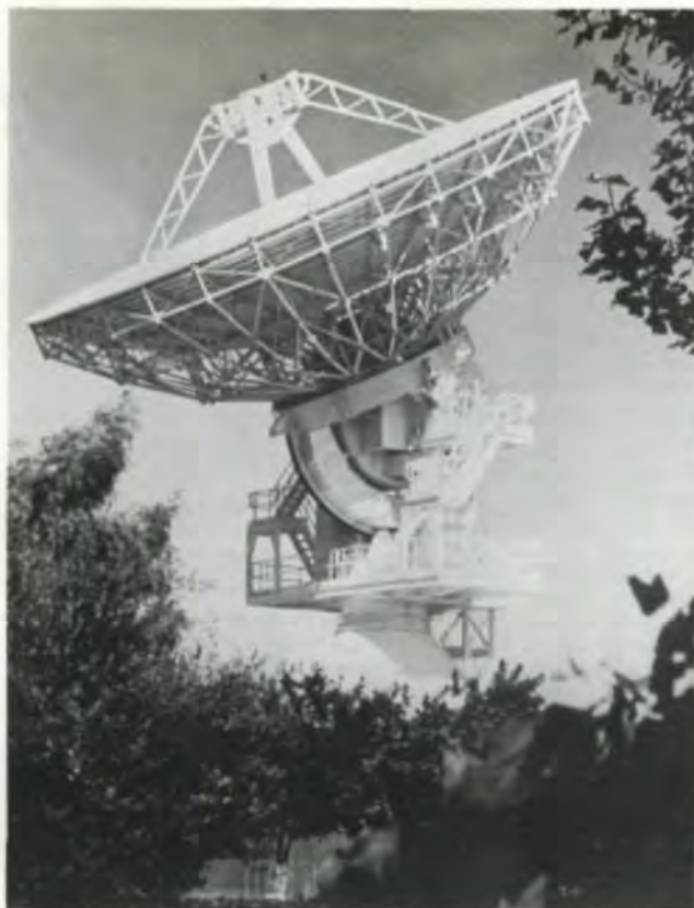
Fig. 8—Microwave antenna with az-el mount.
