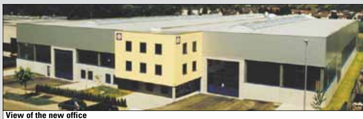
View of the new office
