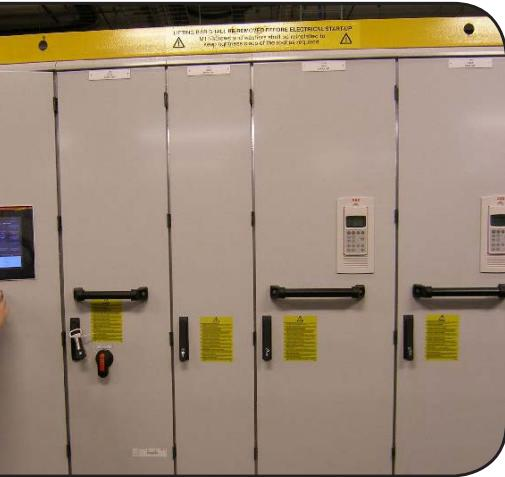
tion problems. ABB's AC500 is also one of the fastest PLCs on the market, and Vard Electro also chose a version of the PLC with one of the fastest processor options—the PM590-ETH—to ensure very good real-time control performance. The PLC is connected to the drive using Profibus DP fieldbus communications.
