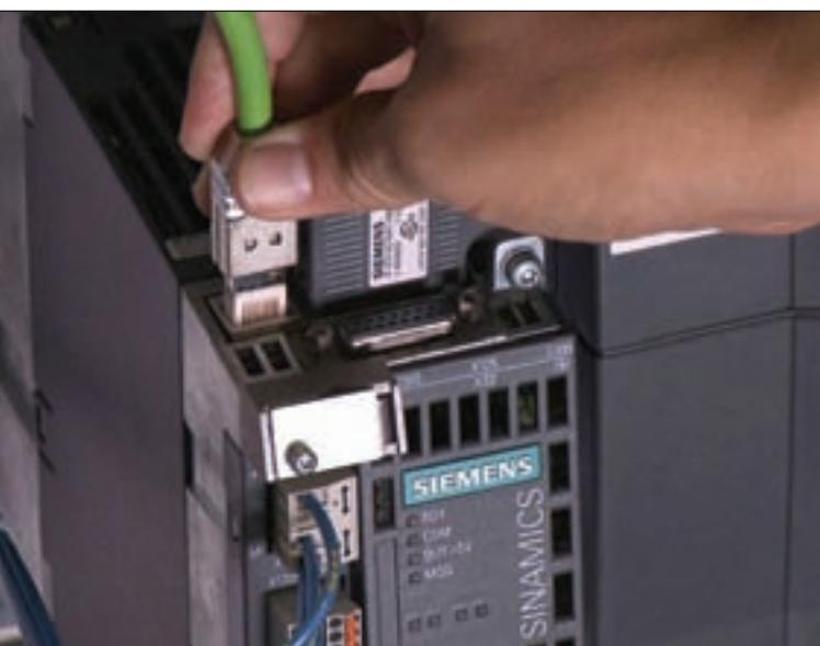
**The Drive-ClIQ connection between motor and drive allows automatic configuration at the motor's power-up, and encoder parameters provide a plug-and-play servo system.**
