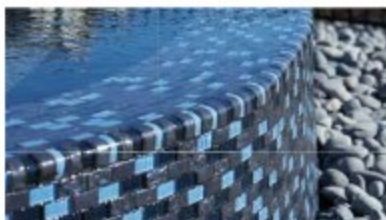
Details Make the Difference. Matching Glass Bullnose Trim Tile available for an attractive finished edge.(as shown)
