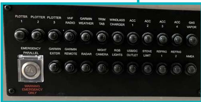
12v Helm Breaker Panel
