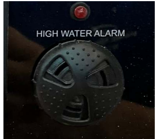
High water alarm
