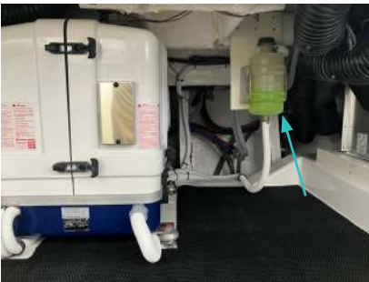
Generator coolant reservoir
