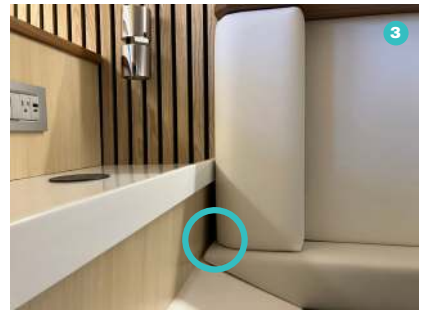
Bottom panel to be removed
