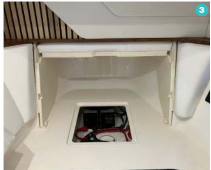
Bow battery access
