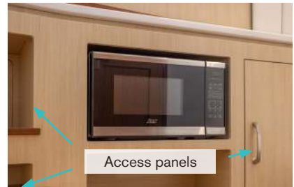
Microwave and access panels
