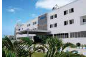
Rudrapur Plant (Green Building)
