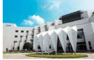
Tainan Plant (Diamond-rated Green Building)
