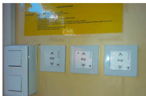
The Somfy io motor is used to operate each of the three blinds in the room independently by wall control.
