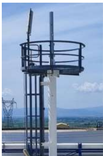
Figure 1. Continuous Vent stack
