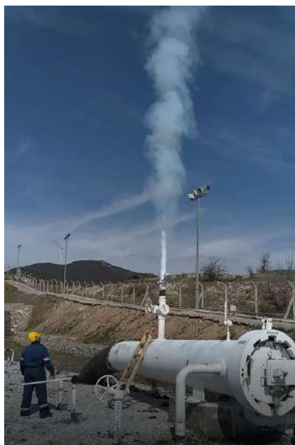
Figure 3. Gas venting during depressurization of a scraper trap.
