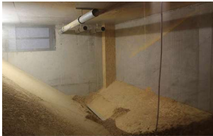
Figure 2. Storage construction for wood pellets (sbz-online.de).
