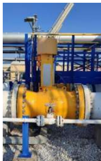
Figure 2. Air operated flow control valve
