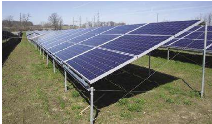
Figure 1. Ground mounted photovoltaic structure.
