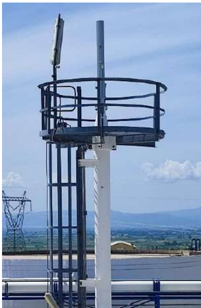
Figure 1. Continuous Vent stack.
