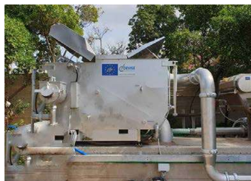
Figure 1. Inlets-outlets of microsieving process (left); Microsieve installed at Rethymno WWTP (right).
