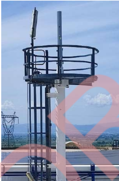
Figure 1. Continuous Vent stack.
