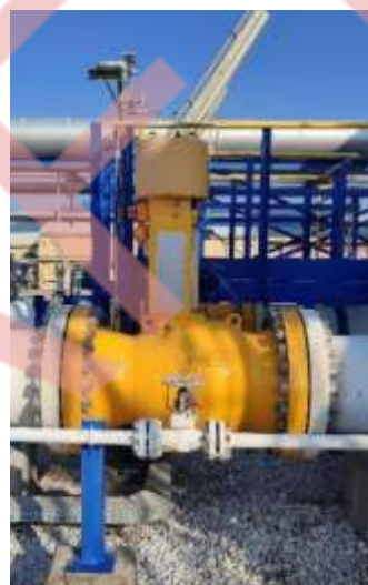
Figure 2. Air operated flow control valve
