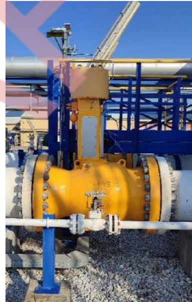
Figure 2. Air operated flow control valve.
