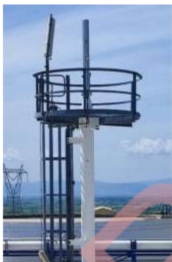
Figure 1. Continuous Vent stack
