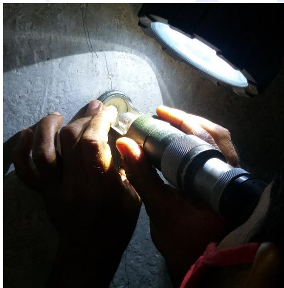
CRACK MEASUREMENT TEST BY MICROSCOPE
