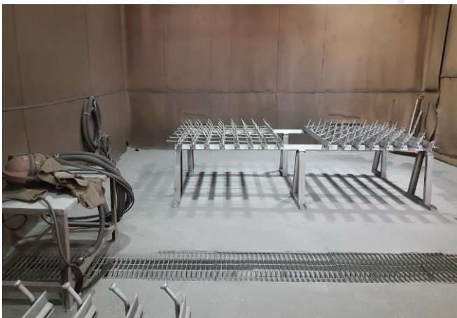
Shot Blast Room
