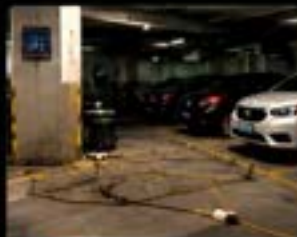
✗ Unsafe grid extensions
