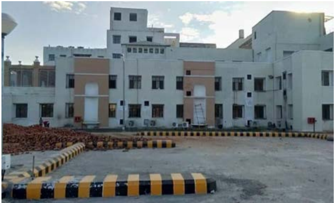
PROJECT- TEZPUR MENTAL HOSPITAL TEZPUR, ASSAM CLIENT- BRAHMAPUTRA INFRASTRUCTURE LTD ELECTRICAL, ELV, FIRE SYSTEMS, NETWORKING
