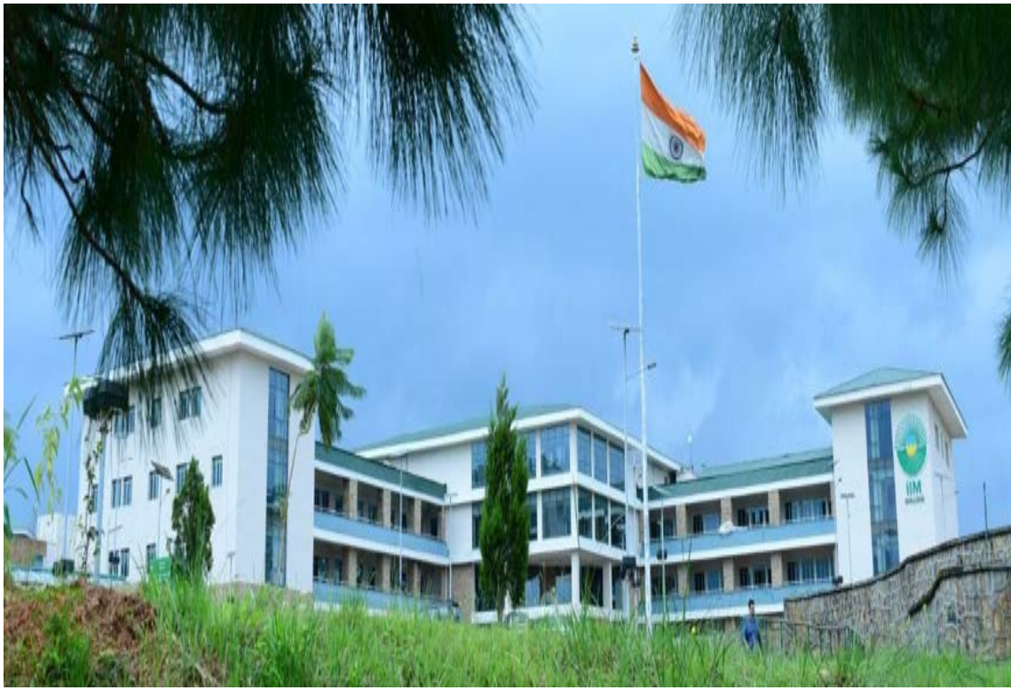
PROJECT- INDIAN INSTITUTE OF MANAGEMENT, SHILLONG ELECTRICAL WORK ( SUB CONTRACT )
