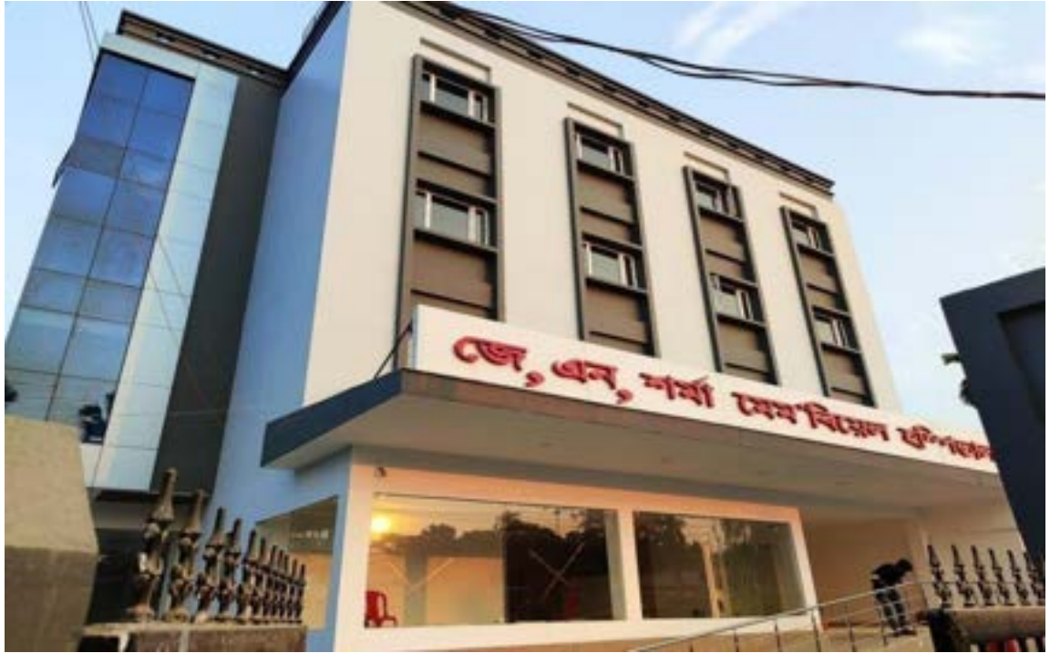
PROJECT- JNSM POLYCLINIC MANGALDAI MANGALDOI ASSAM ELECTRICAL, ELV, FIRE SYSTEMS, NETWORKING
