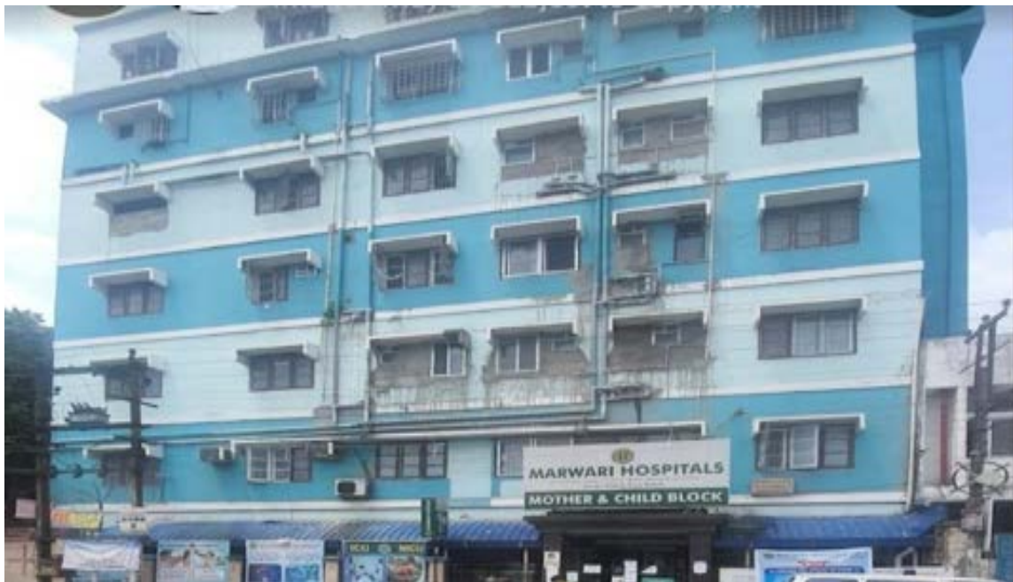
PROJECT- MARWARI HOSPITALS GUWAHATI (INTERNAL RENOVATION WORK) CLIENT- INTEGRA VENTURES STREAMLINING HEALTHCARE (60 BEDDED HOSPITAL) ELECTRICAL, ELV, FIRE SYSTEMS, NETWORKING
