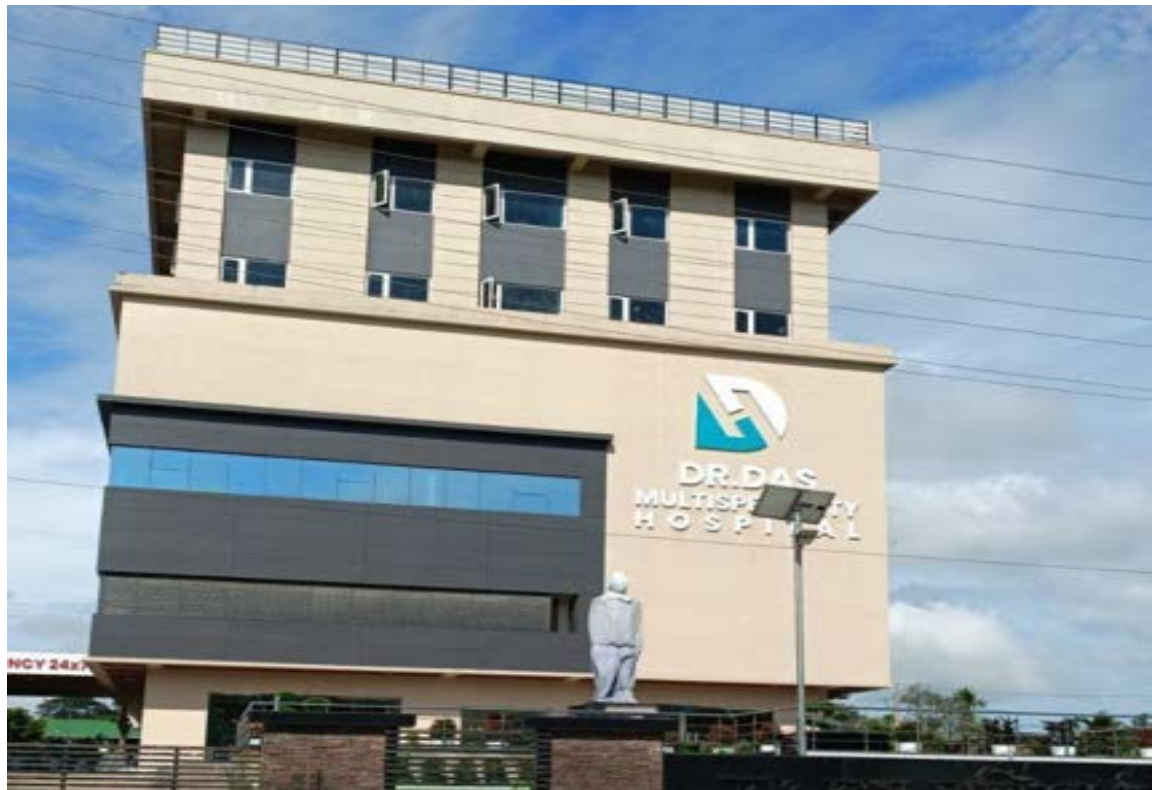
PROJECT- DR. DAS MULTISPECIALTY HOSPITAL NORTH LAKHIMPUR, ASSAM (100 BEDDED HOSPITAL) ELECTRICAL, ELV, FIRE SYSTEMS, NETWORKING
