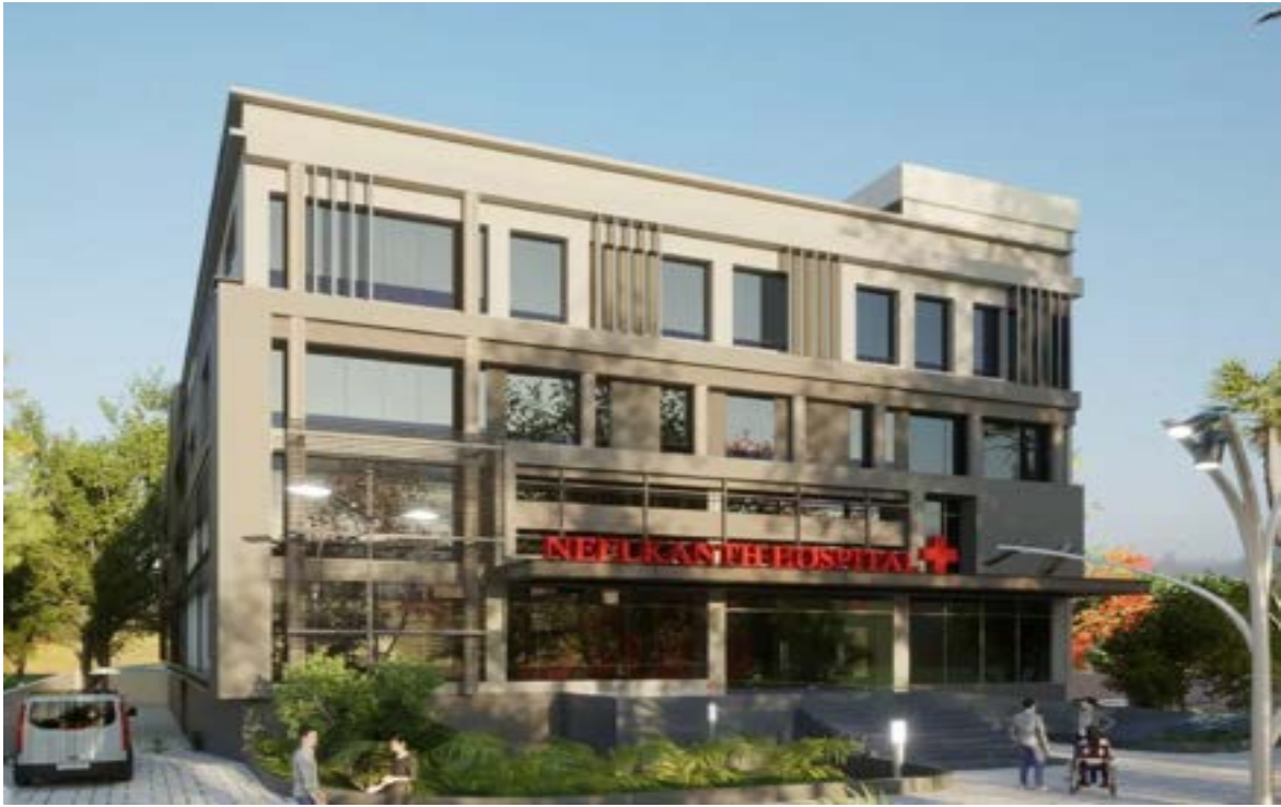
PROJECT- NEELKANTH SUPER SPECIALITY HOSPITAL, TEZPUR ASSAM (200 BEDDED HOSPITAL) ELECTRICAL, ELV, FIRE SYSTEMS, NETWORKING
