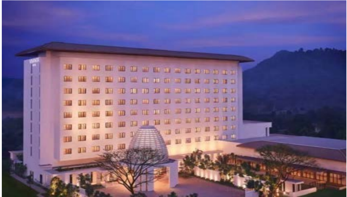
PROJECT- VIVANTA BY TAJ HOTEL, GUWAHATI, ASSAM CLIENT- SHAPOORJI PALLONJI PVT LTD ELECTRICAL, ELV, FIRE SYSTEMS, NETWORKING
