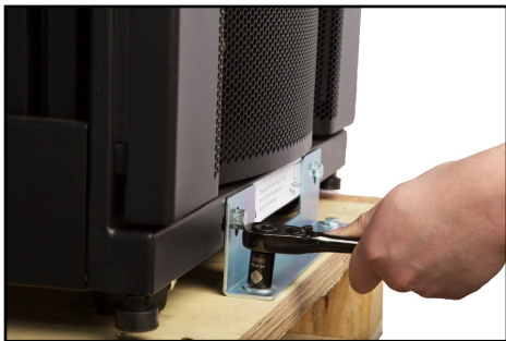
Removing the Bolts
