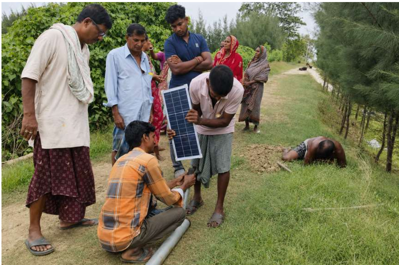
Photo 19: A solar streetlight under installation by a trained local youth at Mandirtala village, Ghoramara Island
