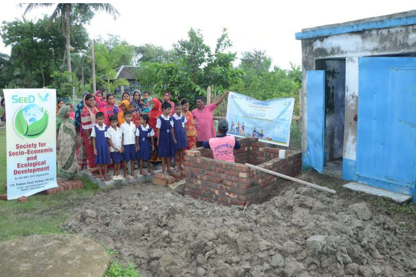
Photo 35: Construction of water reservoir in progress at Ray Para Nimno Buniyadi Vidyalay, Ghoramara Island
