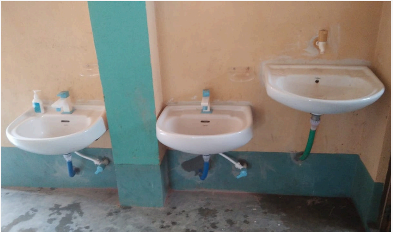
Photo: Wash stations at Multipurpose Cyclone Shelter, Raipara, Choramara
