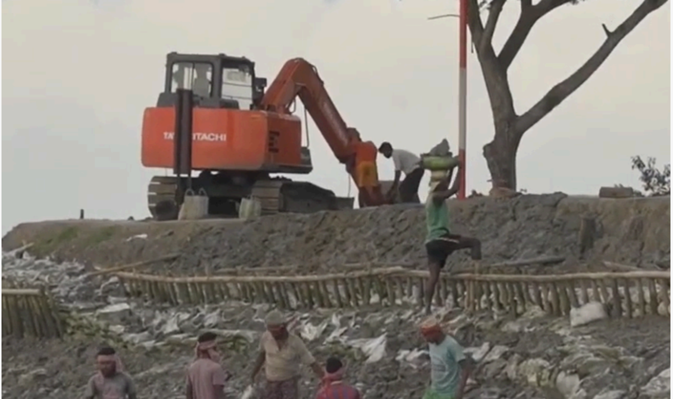
Photo: construction in progress of Multipurpose Cyclone Shelter by involving local labourers
