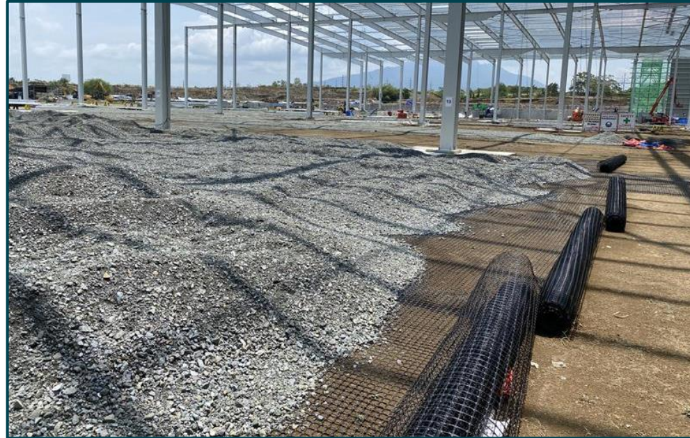
MacGrid EG30S is used in warehouse flooring to improve the mechanical properties of the base course material.
