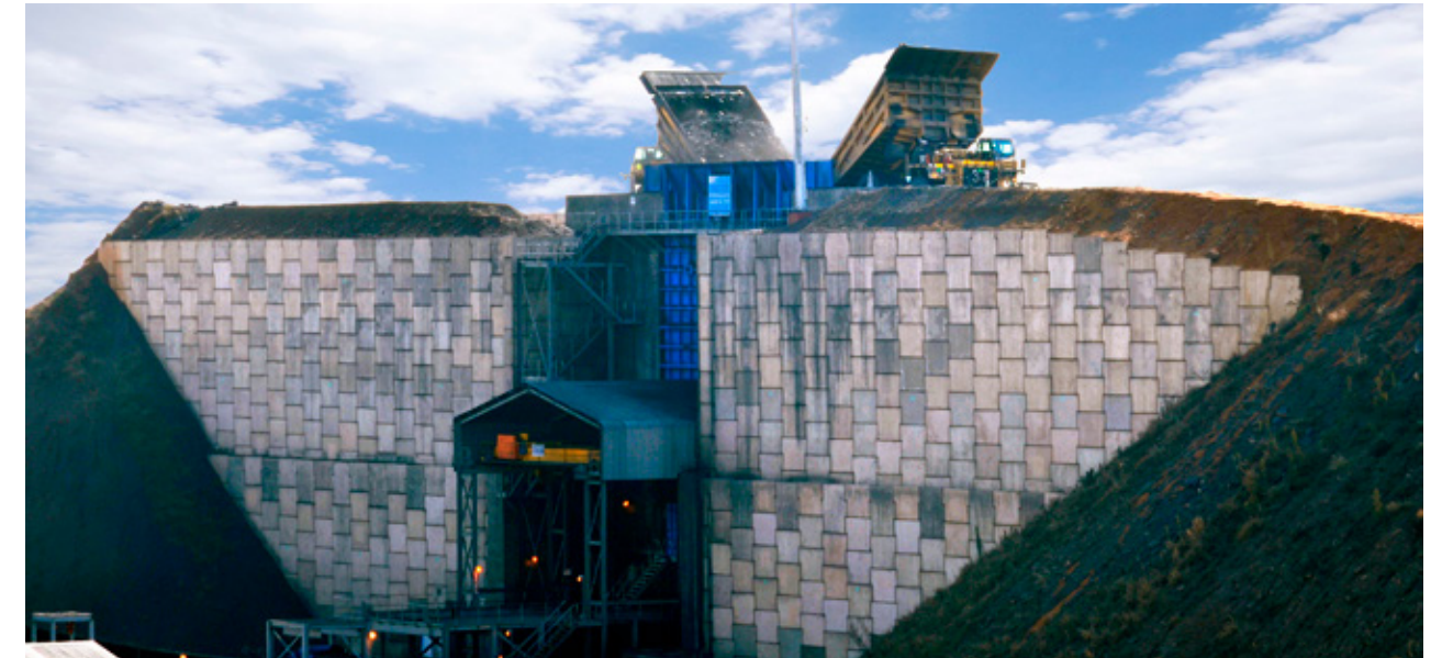
MacRes® concrete faced reinforced soil structure
