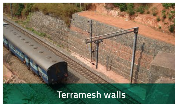
Reinforced soil wall with gabion fascia
