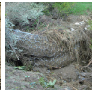
4 Debris Flow & Shallow Landslides
