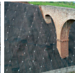
6 Soil Nailing and Surface Protection
