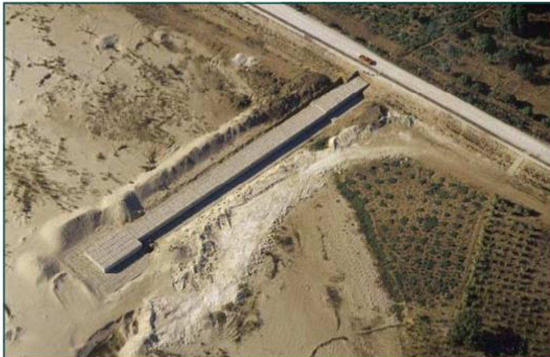
Straight gabion groyne
