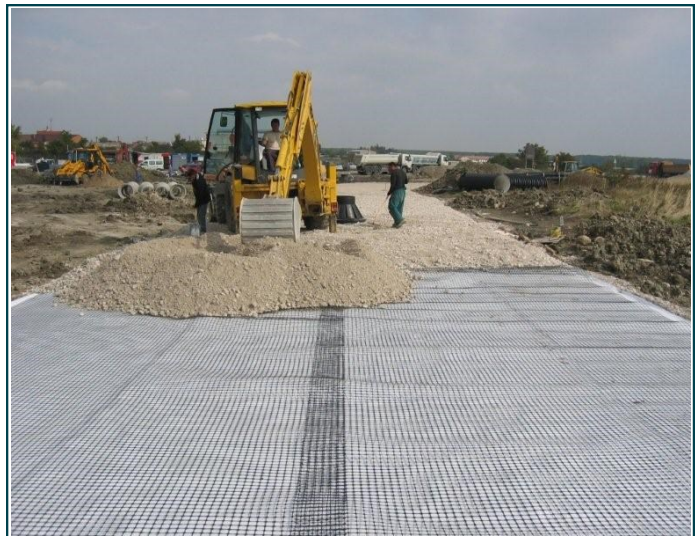
Figure 3 - MacGrid EG S & B installation picture
