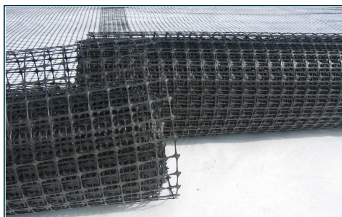
Figure 2 - MacGrid EG S & B installation picture
