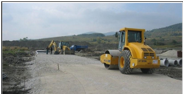
Figure 4 - MacGrid EG S & B installation picture
