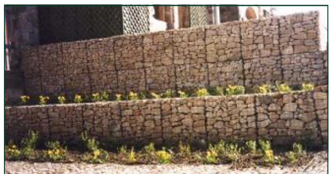
Typical welded gabion installation
