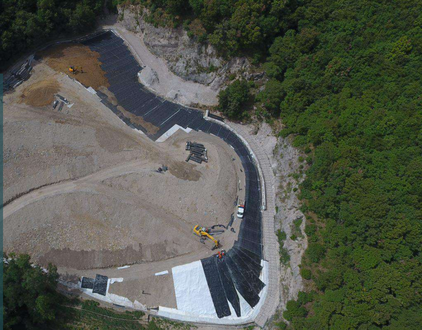
Geosynthetic multicomposite for landfill capping, Cava de' Tirreni, Italy
