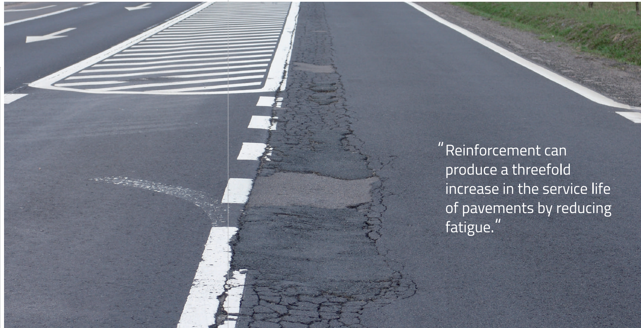
Reinforcing pavements over peat
