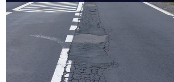
Fatigue cracking
