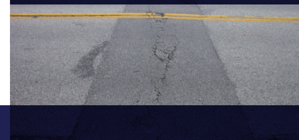
Reflective cracking
