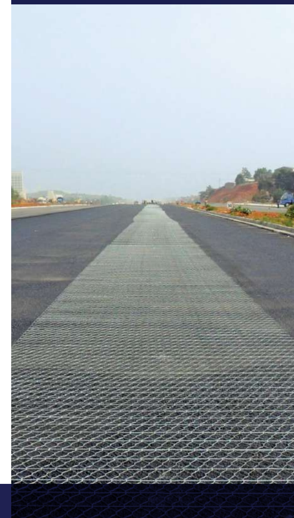
Road Mesh® - Structural reinforcement of asphalt
