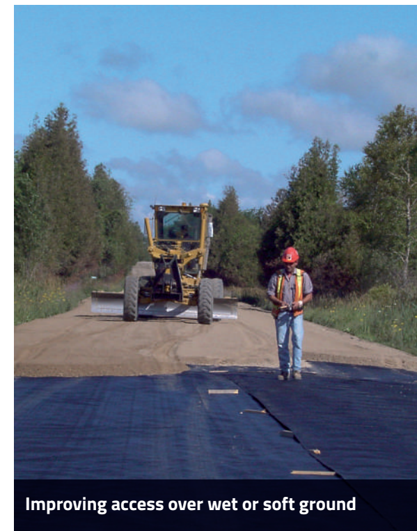
Reinforcing pavements over peat
