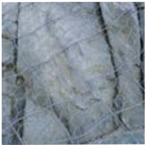
3 Mesh Systems - Secured Drapery / Surface Stabilisation
