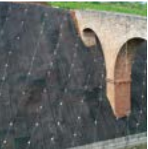
6 Soil Nailing and Surface Protection
