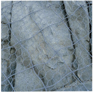
3 Mesh Systems - Secured Drapery / Surface Stabilisation
