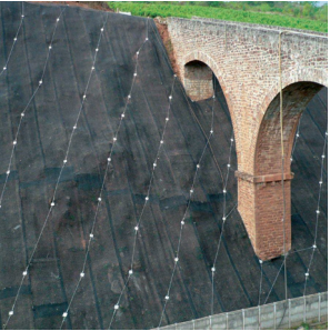
6 Soil Nailing and Surface Protection
