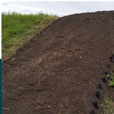
Slope protection with GEOCELLS after backfilling
