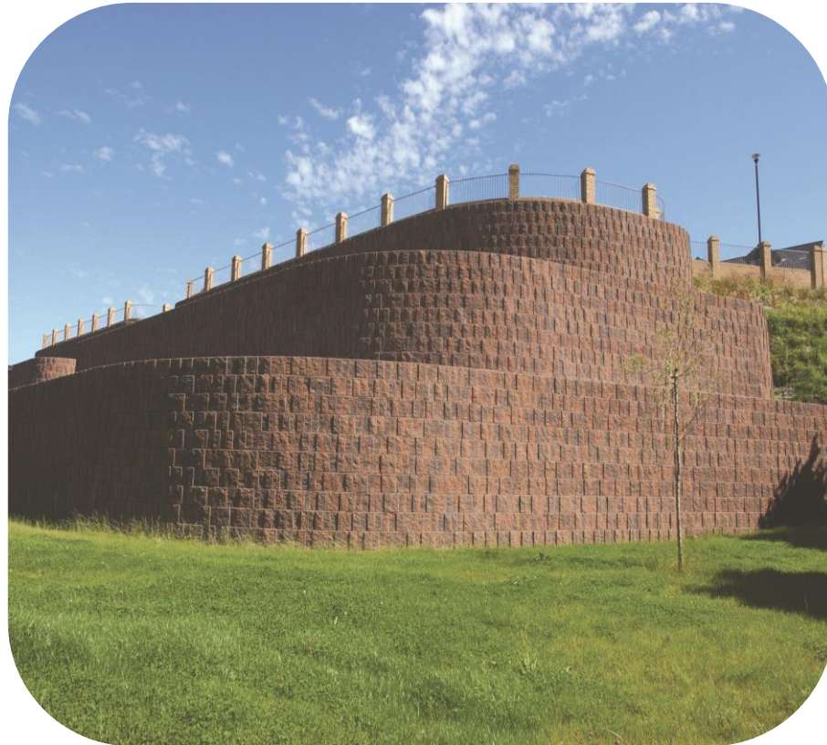
Vertical Concrete Facing with blocks for segmental walls
