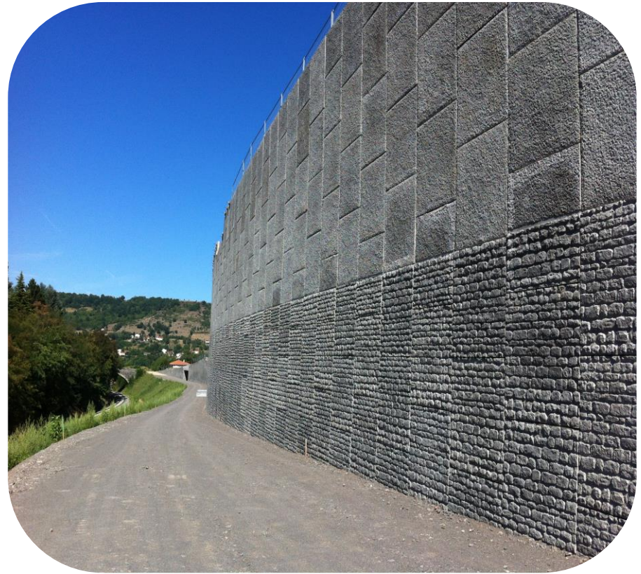
Vertical Concrete Facing with Panels
