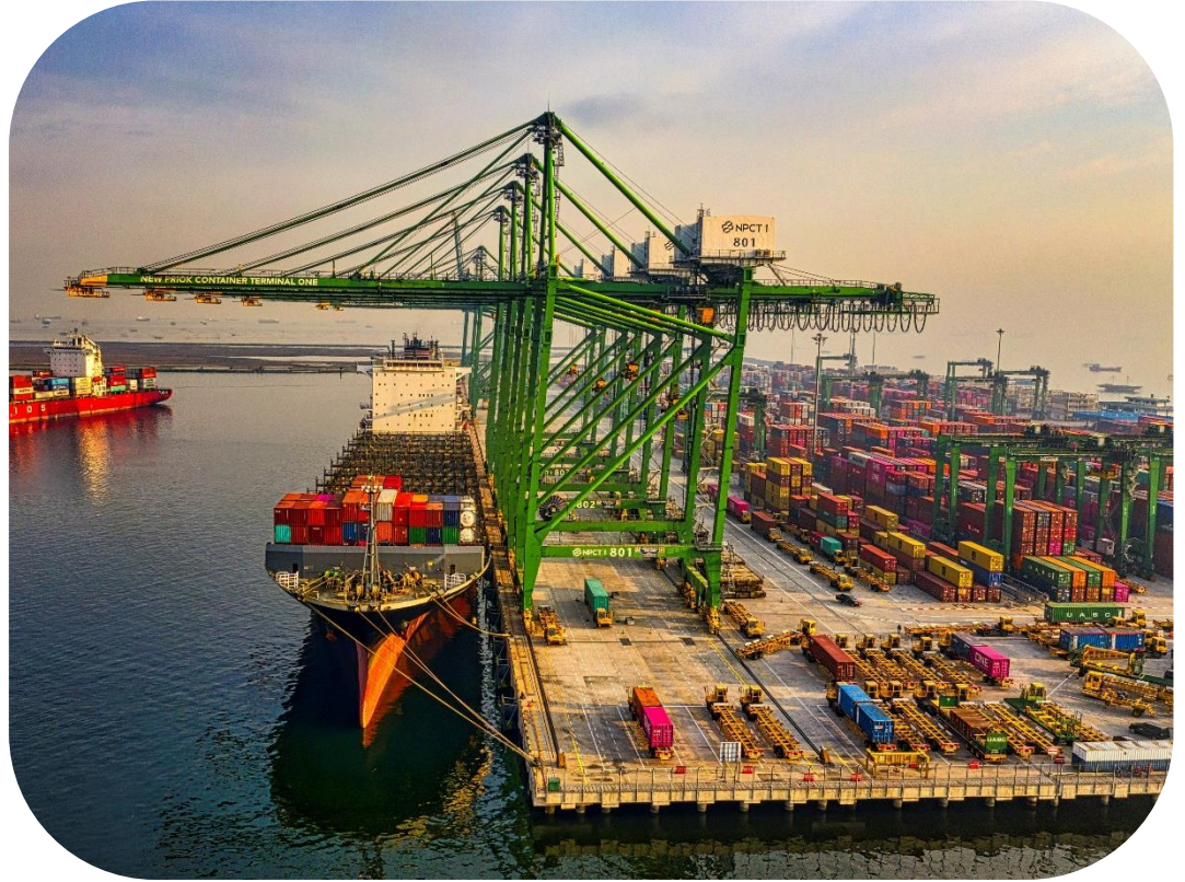
Bottom scour protection in harbor basins
