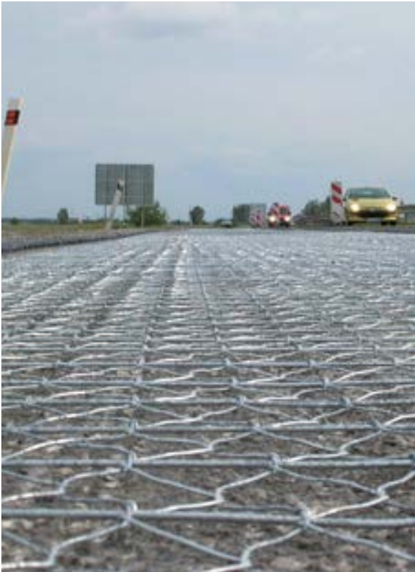
Road Mesh® provides lateral restraint to the asphalt which improves resistance to rutting and shoving
