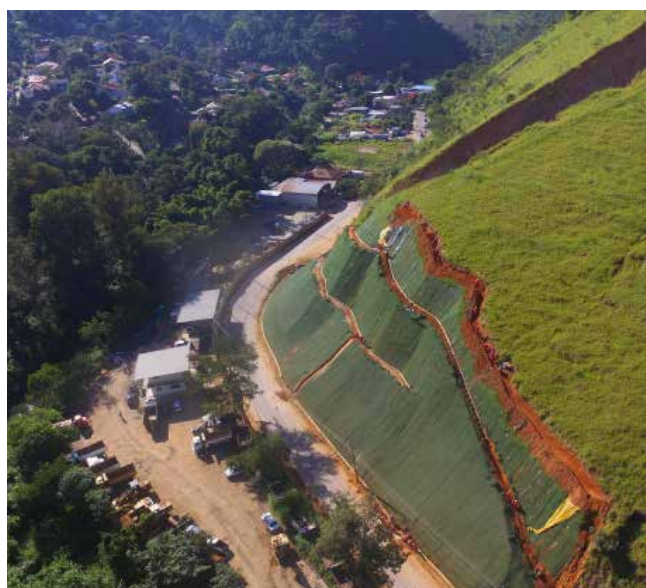
MacMat® R stabilisation of a soil slope face
