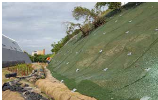
MacMat® R soil stabilisation in industrial park
