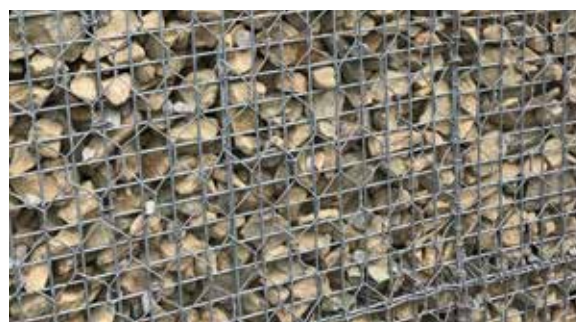
Finished face detail
