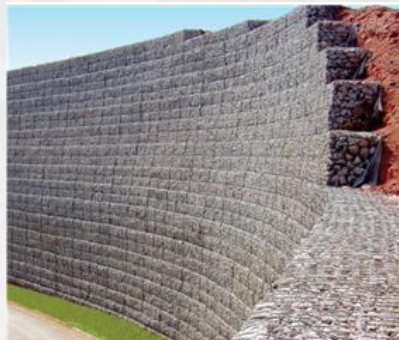
Soil reinforcement with Terramesh® System
