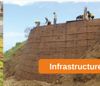
Soil reinforcement with Green Terramesh®
