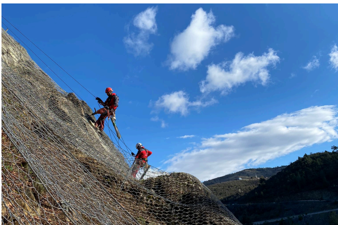
During the construction
