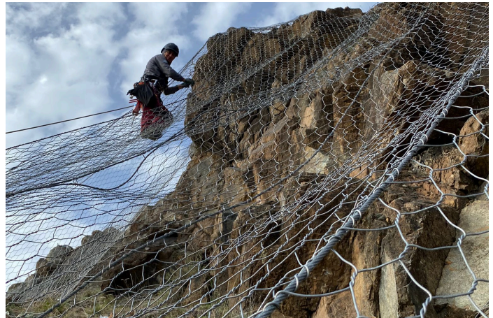
During the construction
