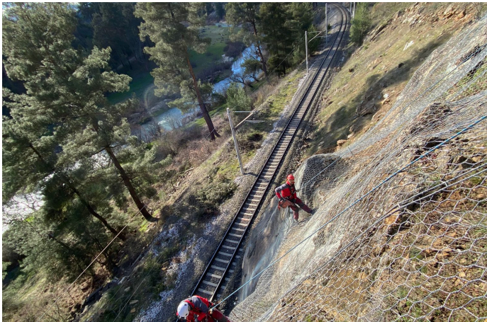
During the construction
