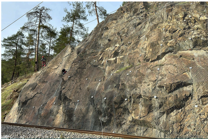
After the installation of HEA Panels
