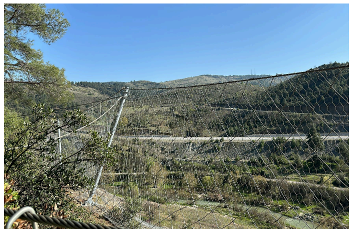
After the installation of dynamic barrier RB 750
