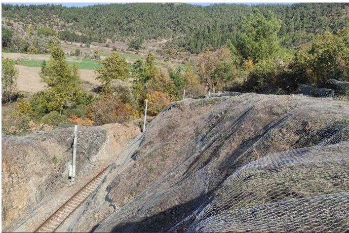
After the installation of HEA Panels
