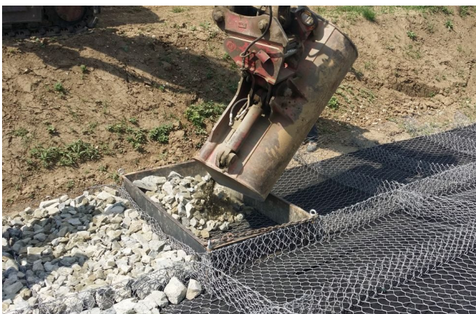
Installation phase: stone-filling operation
