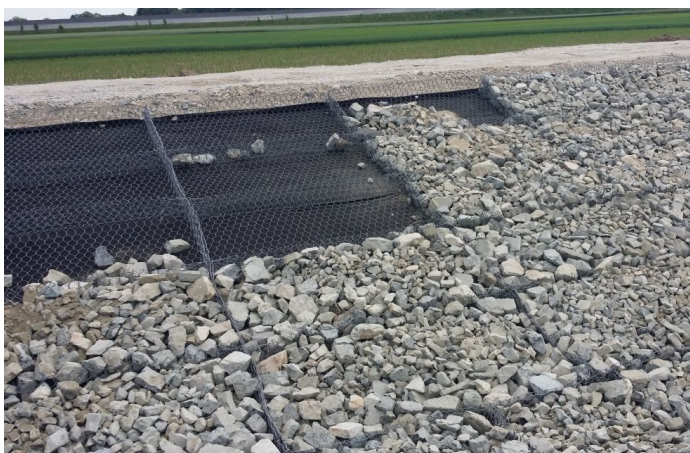
During the installation: stone-filling operation
