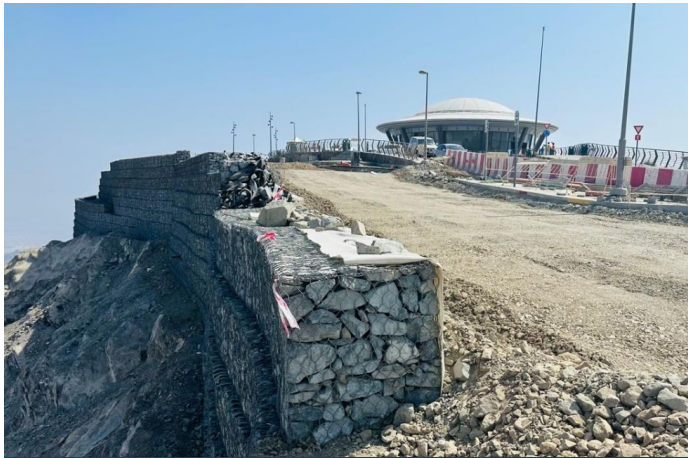
Terramesh wall in progress
