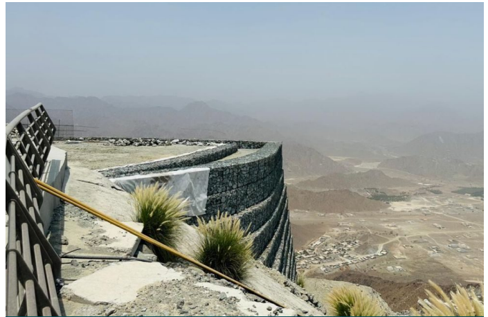
Completed: side view of Terramesh wall
