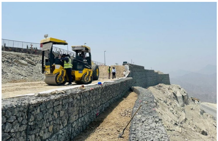
Terramesh wall in progress
