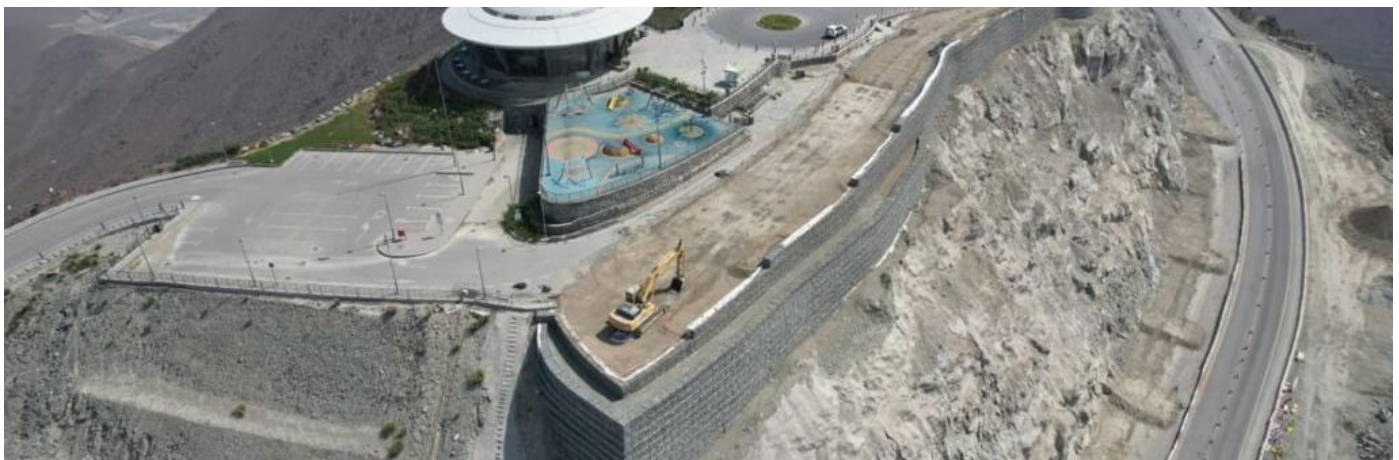
Completed: aerial view of Terramesh wall at parking area
