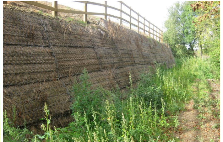
Immediately after construction
