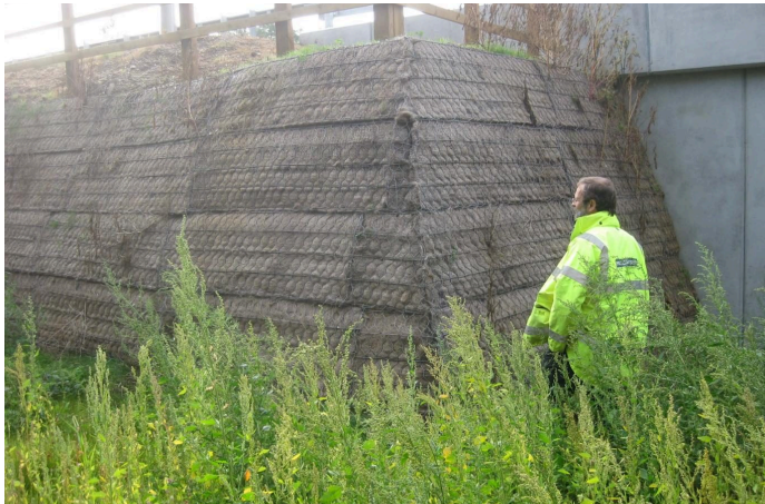
Green Terramesh® Installation after construction
