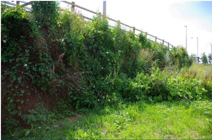
One year after construction
