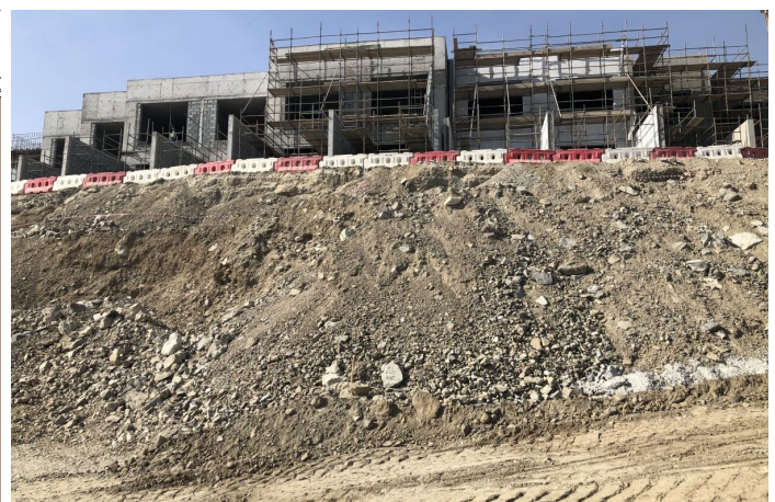
Cut soil slope location for MacWall
