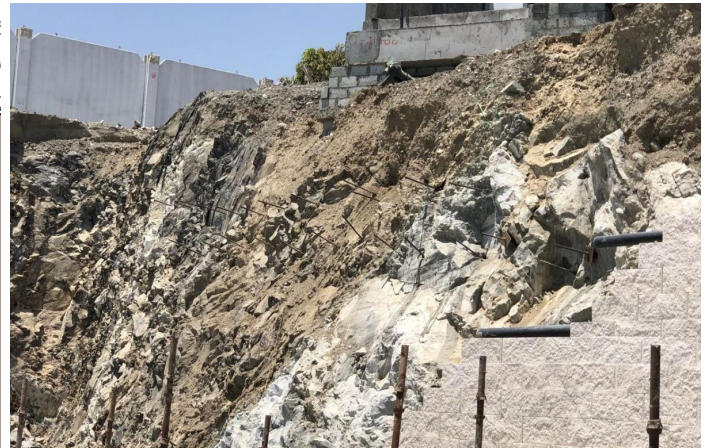
MacWall with rock anchors
