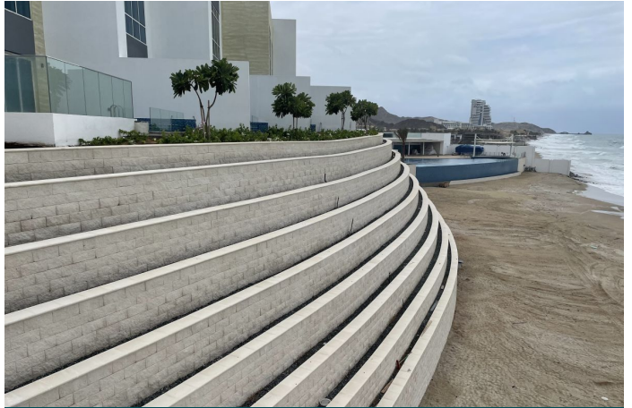
Completed MacWall (tiered details)
