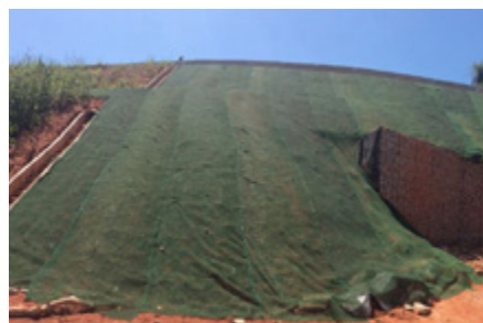
Slope cladding above a retaining wall in gabions with MacMat® R3
