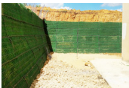
Coating of the face of containments in soil reinforced with MacMat® 10.1
