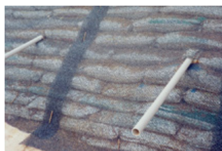
Coating of the face of an erosion recovery with MacMat® 10.1
