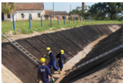
Stormwater drainage channel coating with MacMat® 10.1
