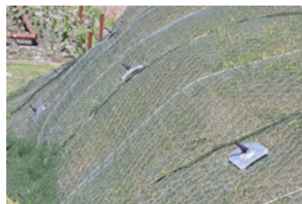
Coating the face of a stapled soil with MacMat® HS
