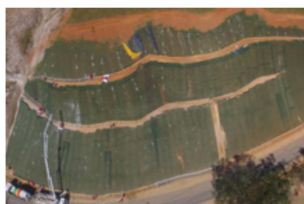
Coating of the face of a soil stapled with MacMat® HS or MacMat® R1
