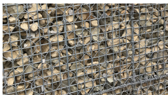
Finished face detail
