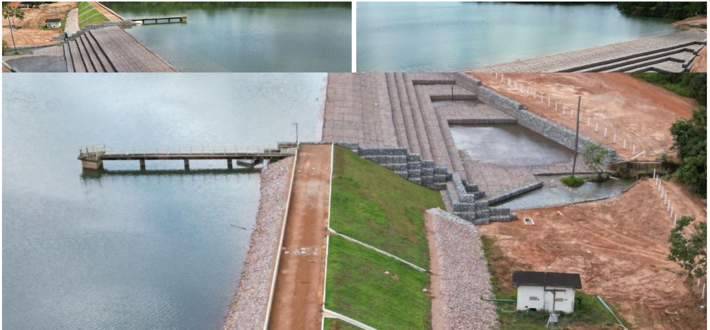
after the construction
