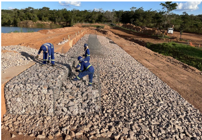
during the construction
