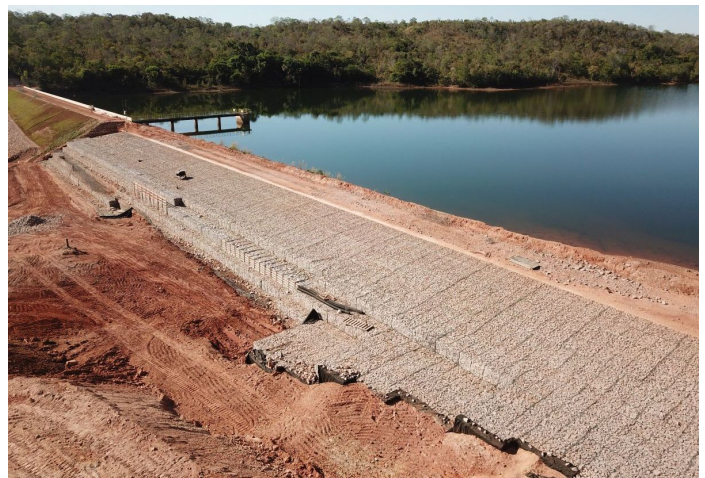
during the construction
