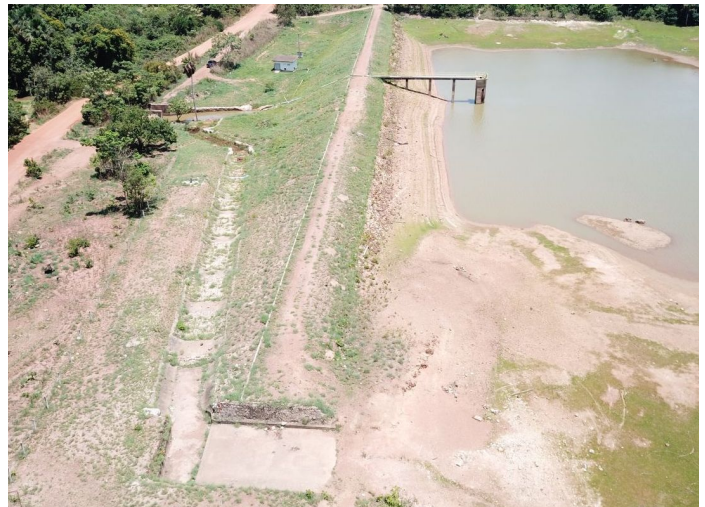
before the construction
