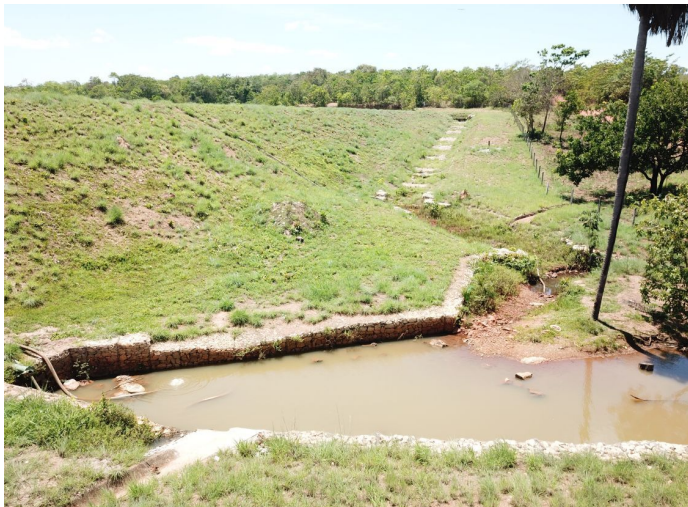
before the construction
