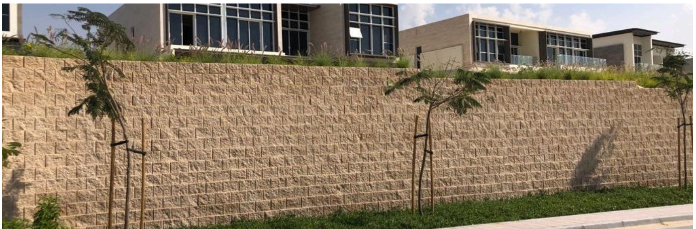
View of completed MacWall with building structure at top
