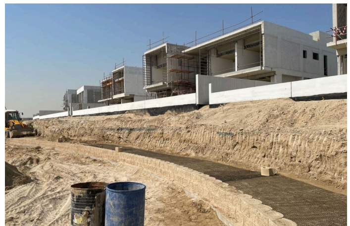
Initial layers during construction
