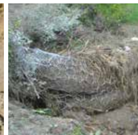
4 Barrera Debris Flow & deslaves.
