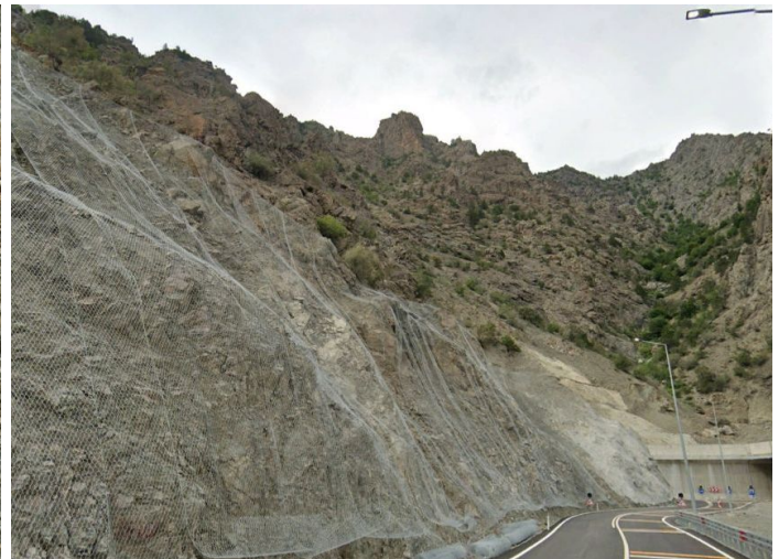
During the construction
