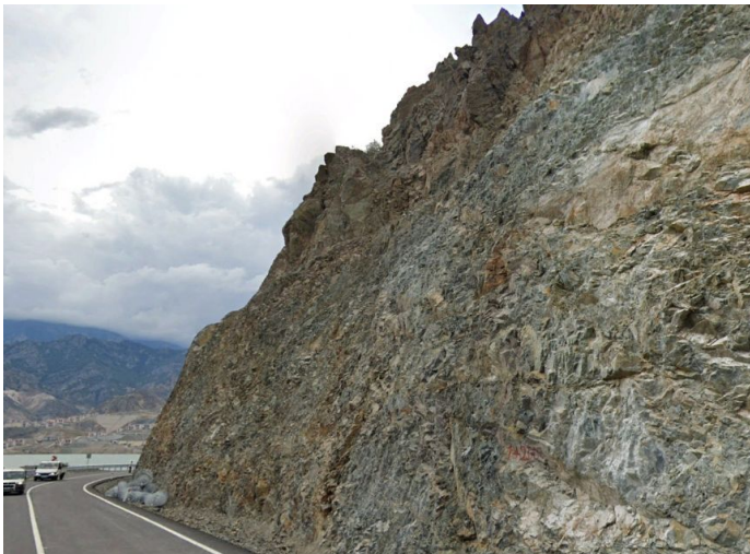
Steep slope outcrop view before drapery system
