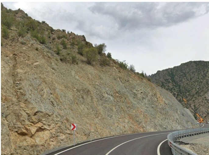
During the construction
