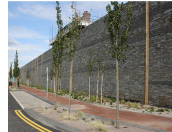
Welded Gabions, BBC Cardiff
