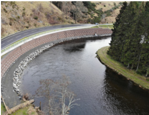
Terramesh® System, A72, Dirtpot Corner
