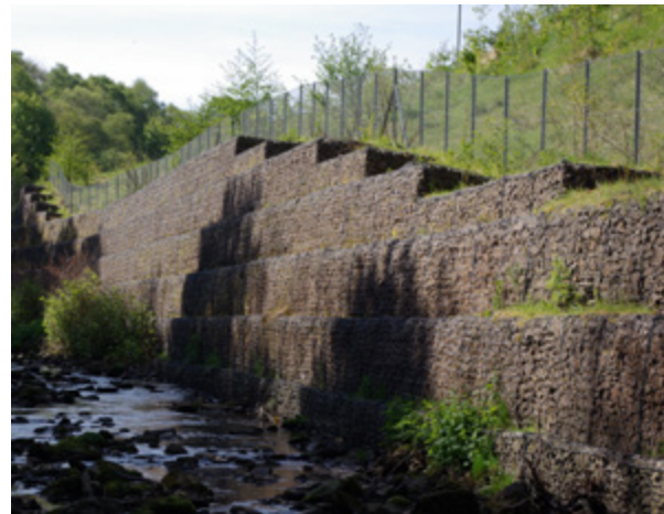
Woven Gabions, Penicuik
