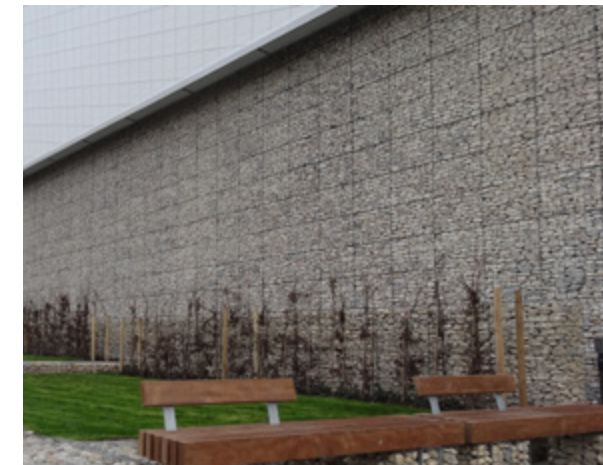
Welded Gabions, Retail Development, Basingstoke
