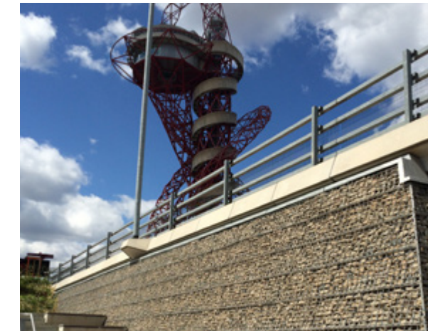
Welded Gabions, Olympic Park
