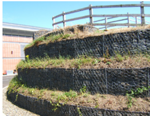
Woven Gabions, Prestwick
