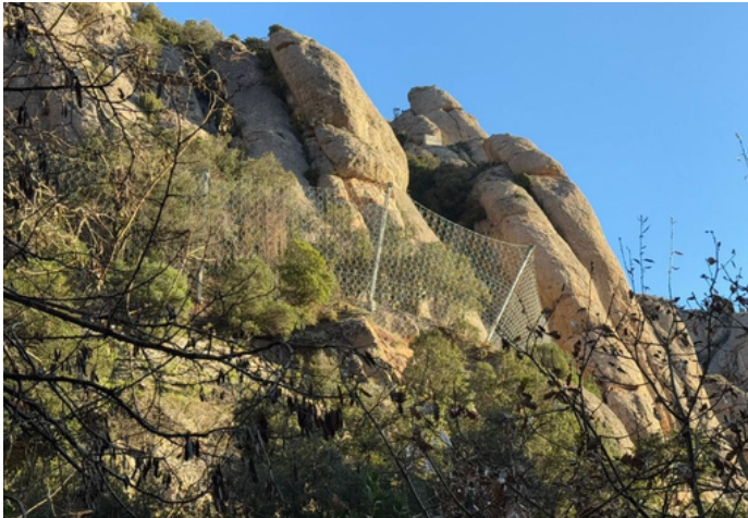
View of the RB 3000 barrier and the slope
