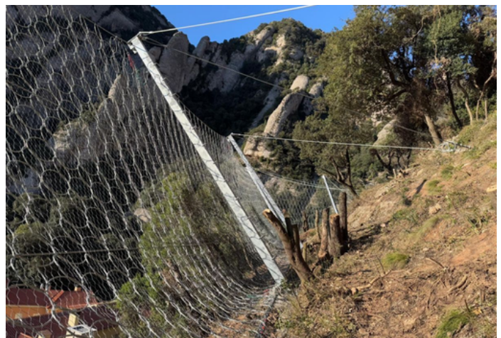
Completed installation of the RB3000 barrier
