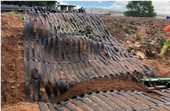
ParaLink® placed in anchorage trench to secure the bond
