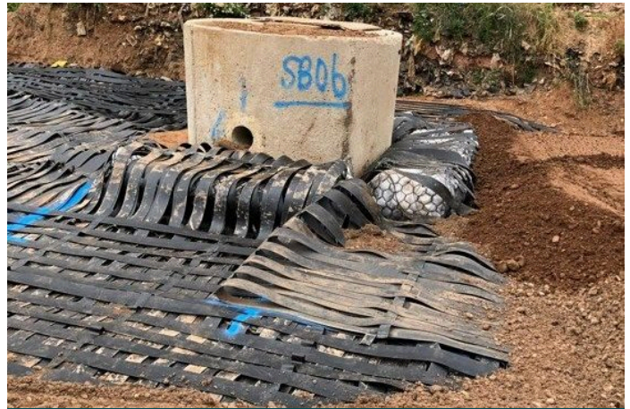
Drainage manhole rings required a gabion thrust block to
