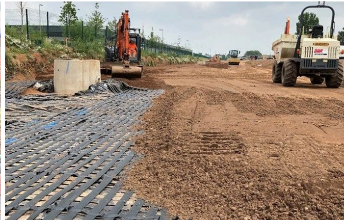
Placement of the granular fill to the basal platform.
