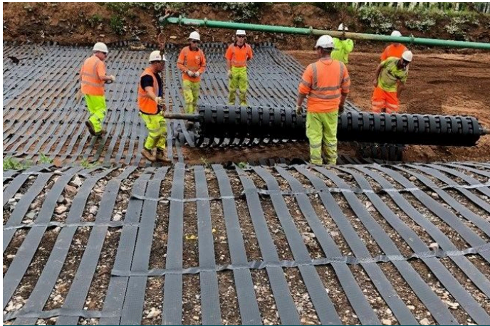
Placement of the transverse layer of ParaLink® with spreader
