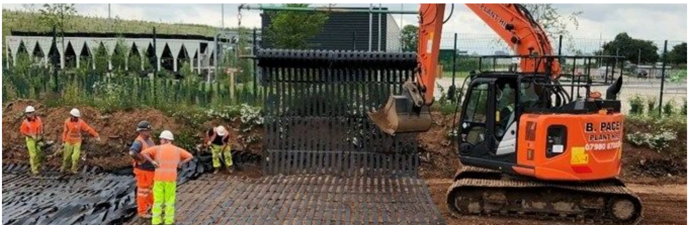
Transverse layer of ParaLink® being installed with a spreader bar.
